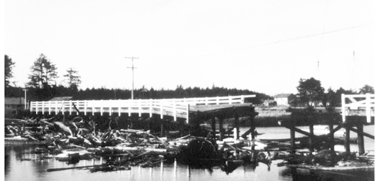
Highway 109 bridge over Copalis River collapsed and trailers and cars were damaged during the 1964 Alaskan Tsunami.
