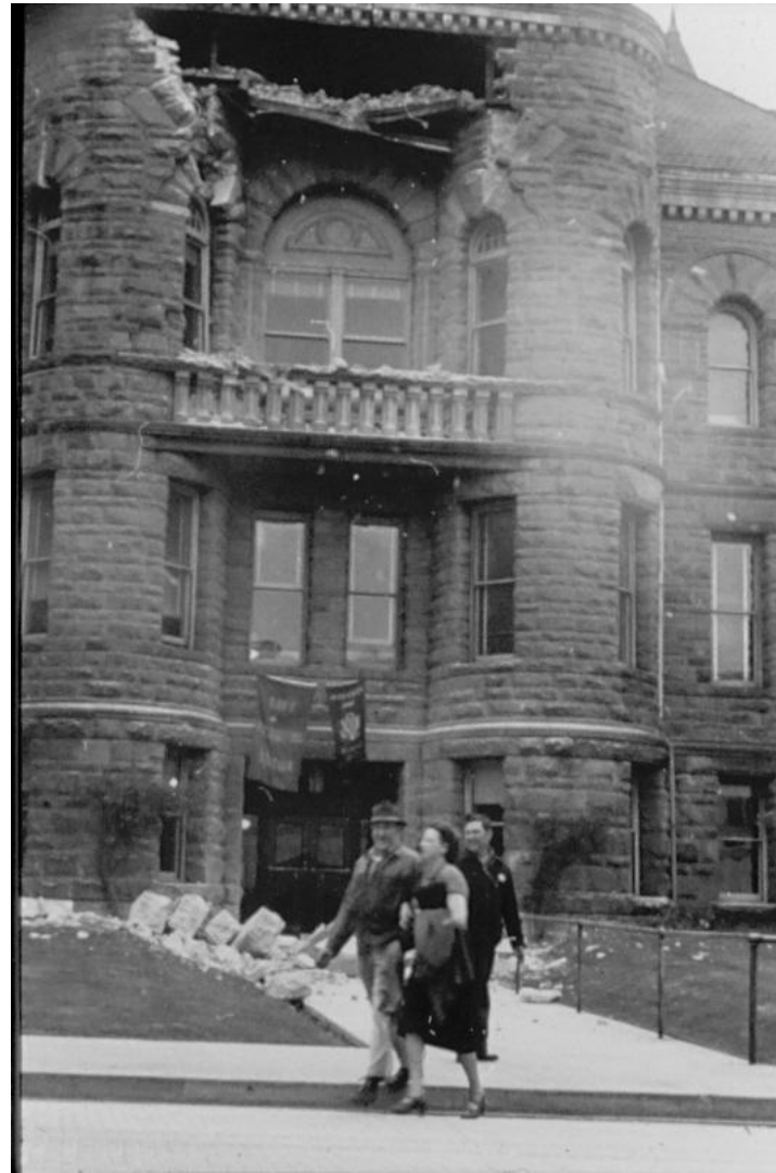
Location 1b. Damage to “old state capitol bulding” in the April 13, 1949 earthquake. Photo supplied by Jim Sims.
