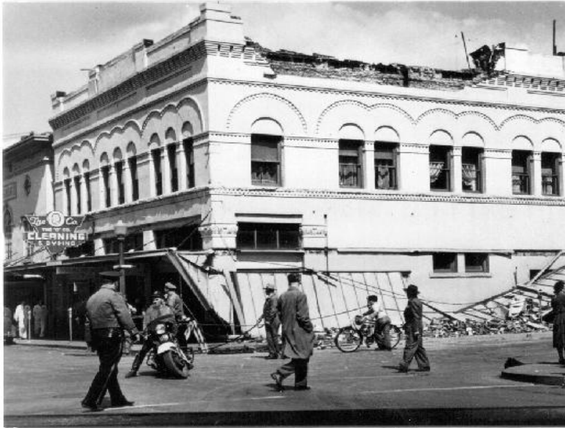
Location 2. Parapet failure in 1949 earthquake, collapsing awning. Although the earthquake occurred at midday on a sunny Wednesday, no one was injured here. Photo by Roger Easton.
