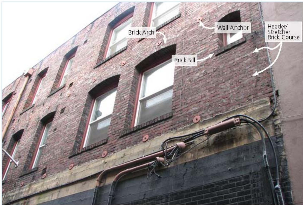
Figure 1. Typical Characteristics of a URM Building.
