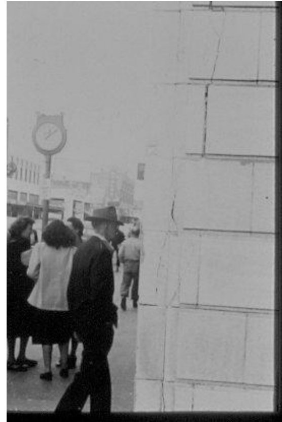
Location 3. Cracking in the wall of the old Capitol Theatre. Photo supplied by Jim Sims.
