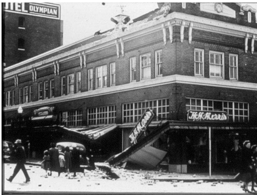
Location 5a. Parapet and awning failure at M. M. Morris, now occupied by Wind Up Here. Photo supplied by Jim Sims.
