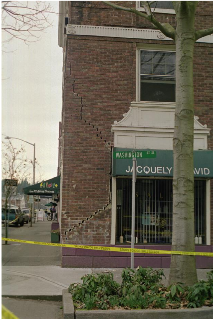
Location 4a. Masonry damage to the Hotel Olympian building in the 2001 Nisqually earthquake. Photo by Josh Logan.
