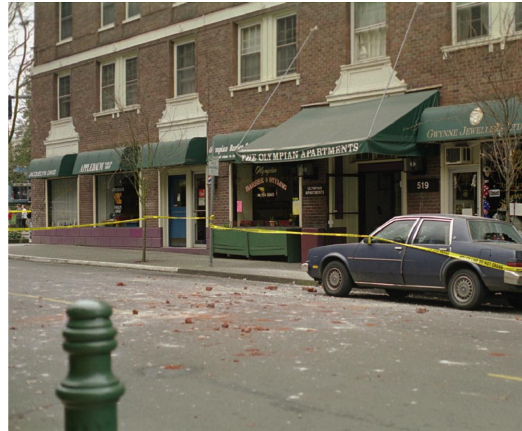
Location 4b. Masonry damage to the Hotel Olympian building in the 2001 Nisqually earthquake. Photo by Josh Logan.
