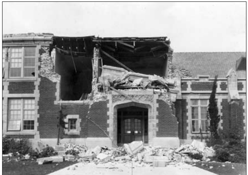
The Long Beach, California school above shows how dangerous old, brick buildings can be. In the 1949 Olympia earthquake, the Senior Class President of Castle Rock High School was killed by falling bricks. The gable on the school collapsed, even though the structure was more than 50 miles (80 kilometers) from the epicenter. Photo: USGS
