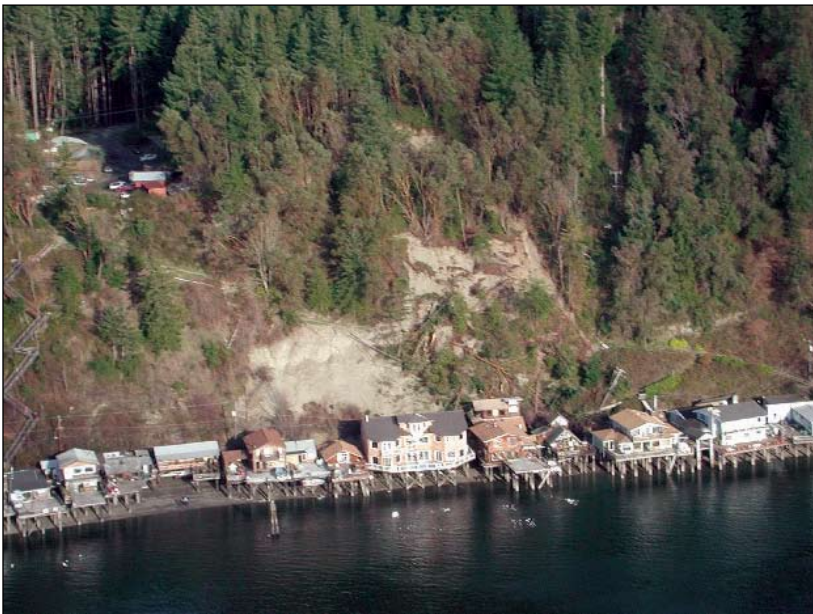
Salmon Beach, near Tacoma, was the site of a landslide three days after the 2001 earthquake. The same hillside slid after the 1949 event. Photo: Dave Sherrod, USGS
