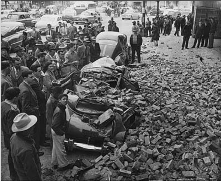
During the April 1949 earthquake, the owner of the Busy Bee Cafe barred the doors to keep panicking patrons from rushing outside. Seconds later, brick fell from the top of the Hotel Seattle, crushing several cars. Photo: Seattle Post-Intelligencer Collection, Museum of History & Industry; All Rights Reserved
