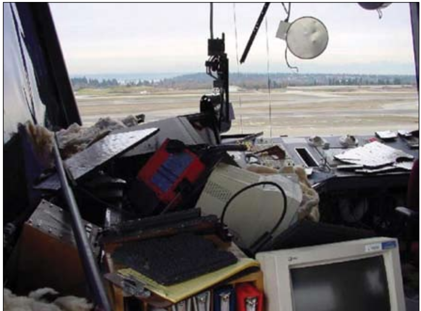
The tower at Sea-Tac sustained both structural and nonstructural damage. Even so, the airport was able to reopen after a few hours. Photo: Washington State Department of Transportation
