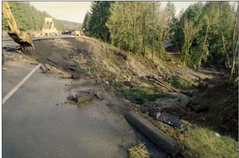
Liquefaction, lateral spreading, and landslides damaged many roads throughout the area. Photo: William S. Lingley, DGER
