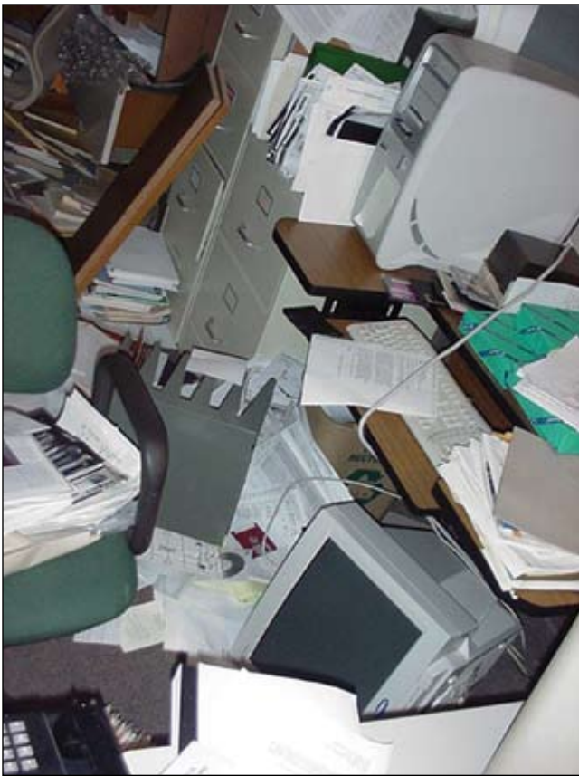
Nonstructural damage in homes and offices, like bookcases, computers, and dishes falling, can be dangerous and expensive. Photo: Ray Lasmanis, DGER
