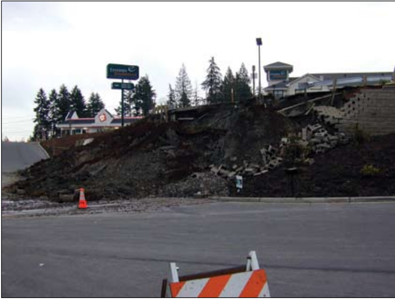
Liquefaction and landslides can break utility lines as well as damage roads and property. With widespread damage, repairs may take longer than expected. Photo: Robert J. Reid
