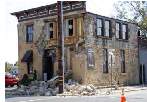
Napa earthquake damage to a building without seismic retrofit
