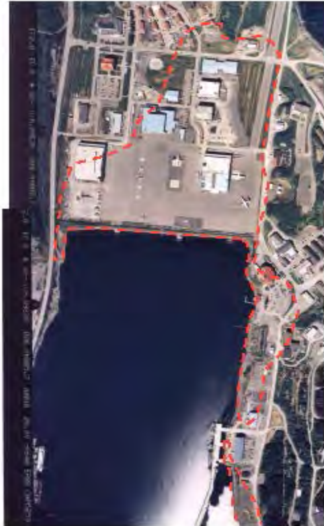
Figure 7. Hydraulic fill (dashed red lines) at the upper end of Womens Bay.
