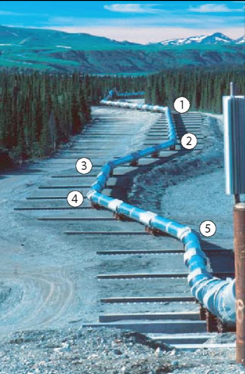
The Trans-Alaska oil pipeline survived the 2002 M7.9 Denali Fault earthquake. Pipeline design accommodated 14 feet of horizontal and 2.5 feet of vertical motion.
