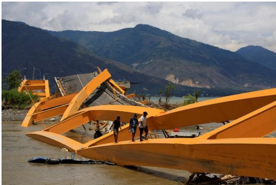
Image: bridge destroyed by the earthquake and tsunami that struck Palu Source: Beawiharta Beawiharta/Reuter
